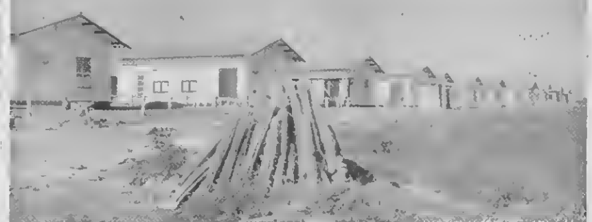
The five-room HBF houses now under construction at Sabaneta will be similar to those pictured above. Although they aren't HBF houses, those above were built by Aruba Construction Company, one of the contractors working on the new group of houses for Lago employees.
